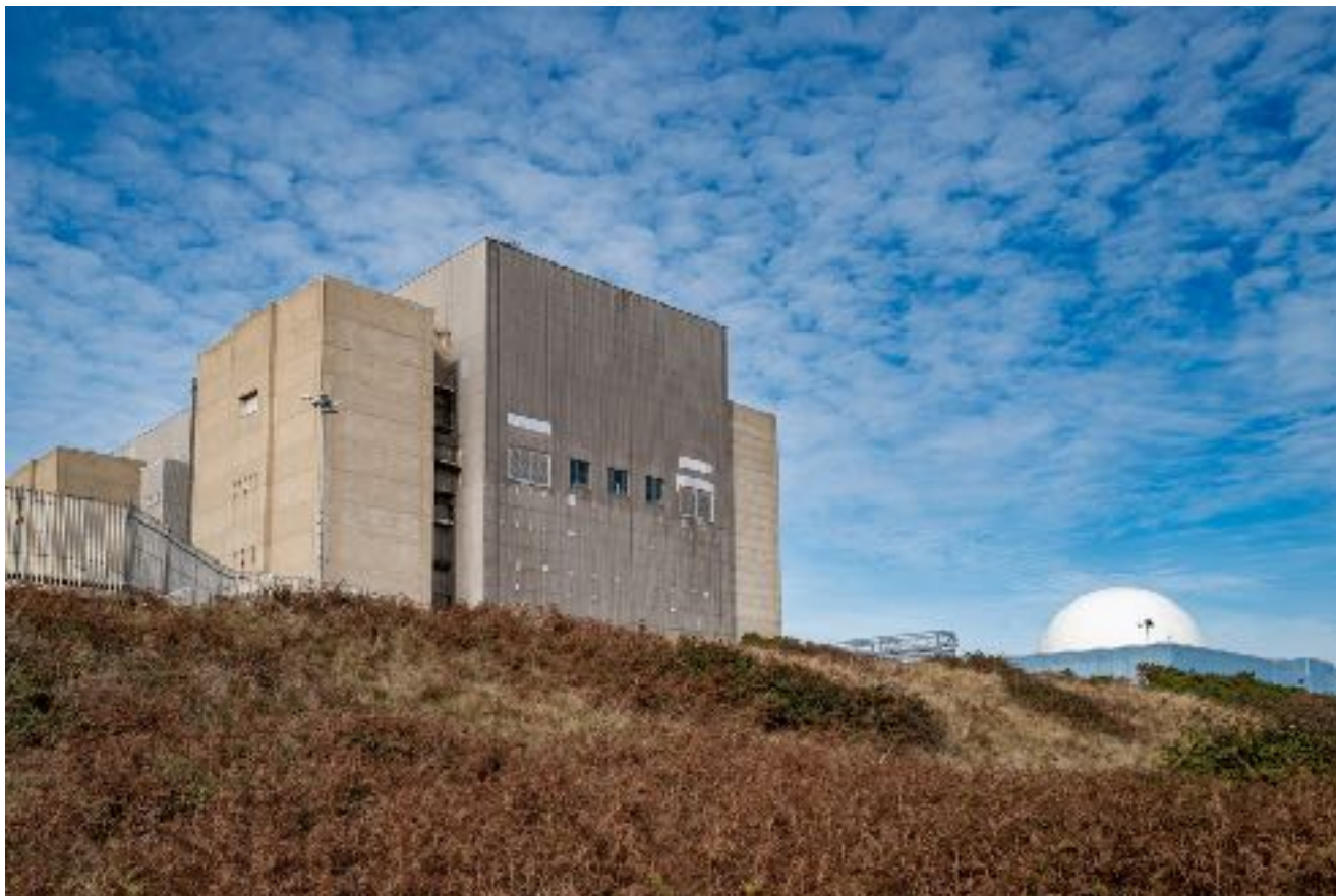
Sizewell A, now decommissioned, was a Magnox station with two reactors of far less than 300MW. In the background is Sizewell B, a PWR with an output of 1,200MW. Scaling up didn't make nuclear economical.
